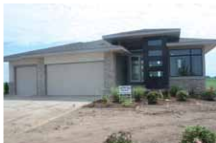
Jerry Bussanmas Homebuilders, LLC
